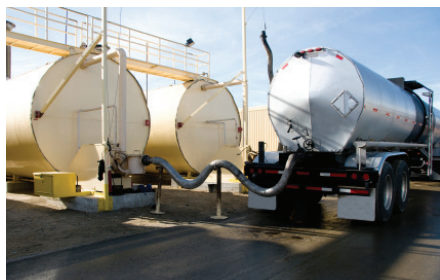
Tank truck unloading.
